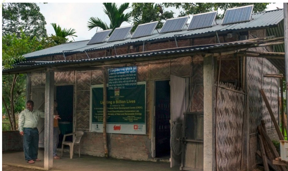
Distributed Solar PV system for rural electrification
